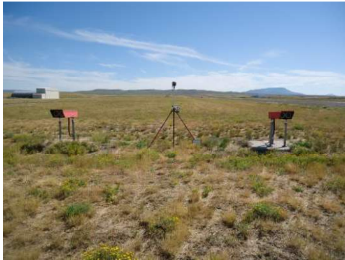
Figure 3.27 Precision Approach Path Indicator (PAPI)
